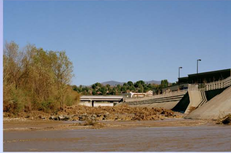
Concrete bank stabilization
